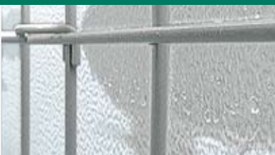
2.) Frost build-up is thawed during auto-defrost
