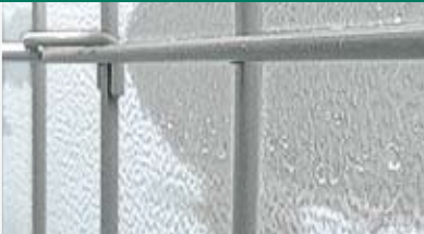
2.) Frost build-up is thawed during auto-defrost
